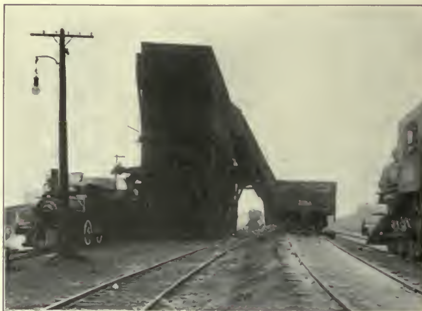
FIG. 666. FACILITIES TO BE ABANDONED. Locomotive coaling station of the Chicago, Rock Island & Pacific Railway, near 47th Street and Armour Avenue. This station has a storage capacity of 500 tons. An inclined belt-conveyor carries the coal from the receiving hopper to the storage bins. In the event of electrification, the structure would be rendered worthless.
